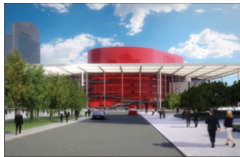
When completed, the performance space will be clad in vibrant red glass, earning the nickname "The Red Drum." A massive solar portico radiates from the building. (Photo: Jeffrey Buehner)
